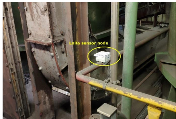
LoRa sensor node in an industrial environment (©Lakeside Labs GmbH)
